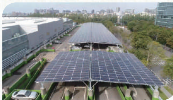
Parking tower at Si-Soft Research Center
