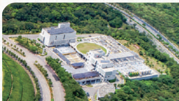
Tongluo Science Park sewage treatment plant
